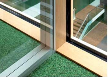
A special profile ensures flexible mounting of the adapter on the façade whilst maintaining the high level of sound proofing. This enables the user to reposition the walls within the building whenever necessary.
