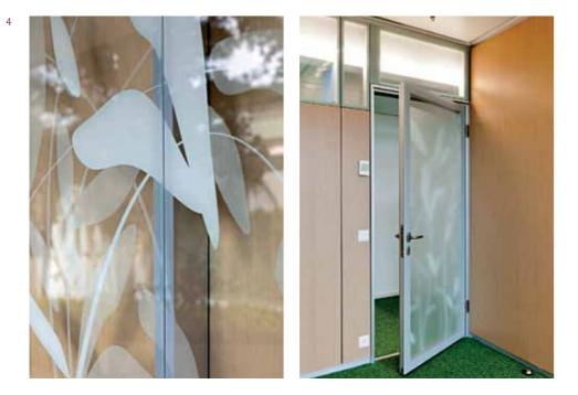
The floral print over doors and corner elements creates the impression of one continuous flowing space. The special foil coating on the toplight glazing evenly distributes the strip lighting.
